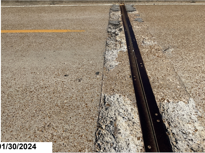
Spalls with rebar exposed with s/l to deck @ end of Span 9. (#3)
