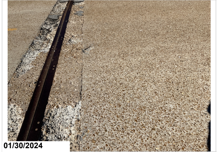
Spalls to deck @ beginning of Span 10.(#3)
