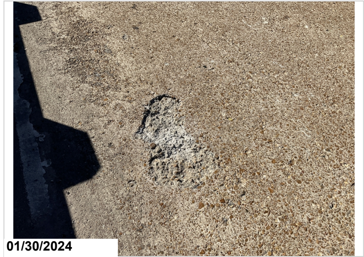
Spalls to deck @ Span 1.(#3)
