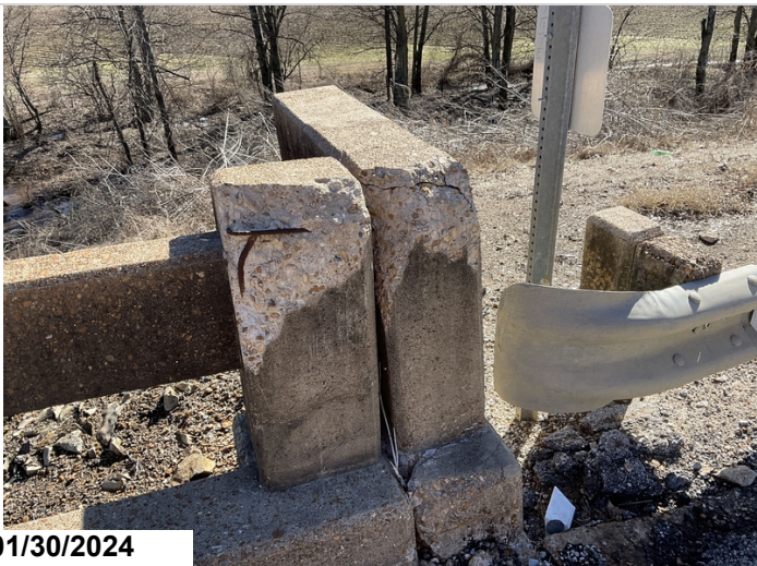
Damage to Right end post & Post 1 on Right @ Abutment 1. (#3)
