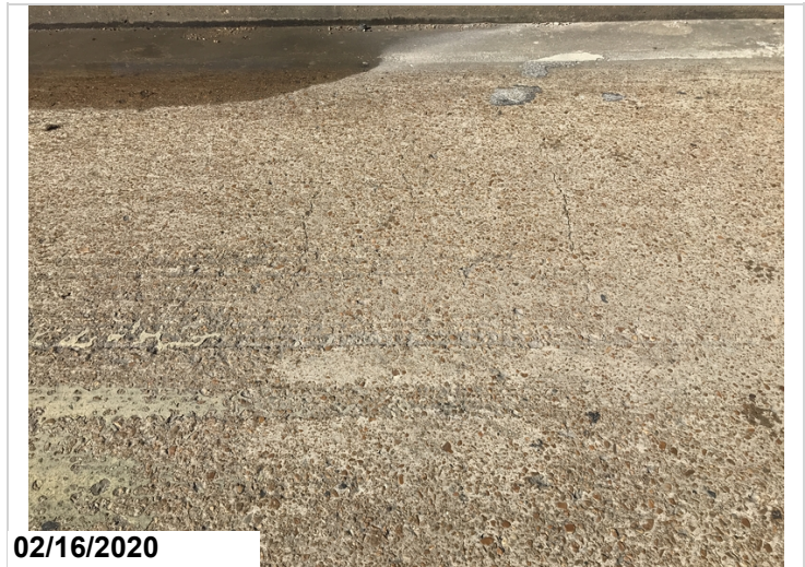
Transverse cracking to deck @ Span 1.(#3)
