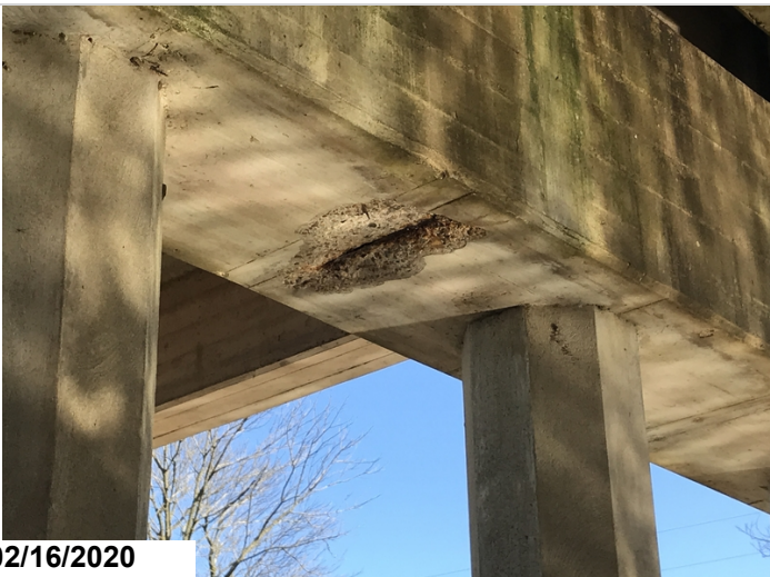
Spall with rebar exposed with s/l to bottom of cap @ Bent 5. (#3)
