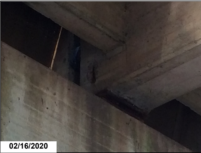
Spall w/ 4" rebar exposed to Girder 2 at beginning of Span 6
