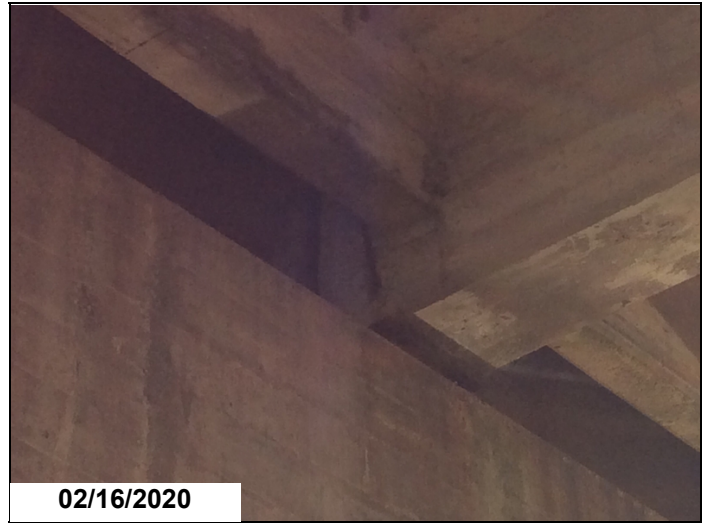
Spall w/ 1' rebar exposed to Girder 3 at end of Span 5.
