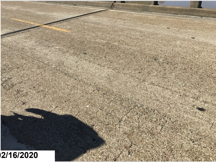
Transverse cracking to deck @ Span 11.(#2 & #3)
