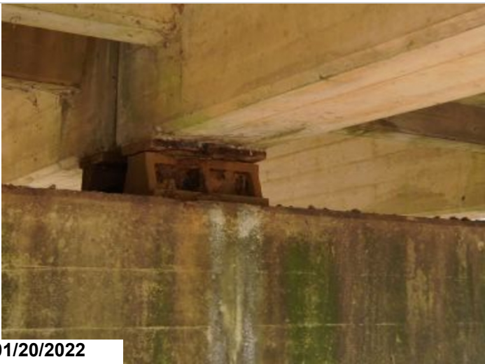
Missing anchor bolt to Girder 2 backside of Bent 2.
