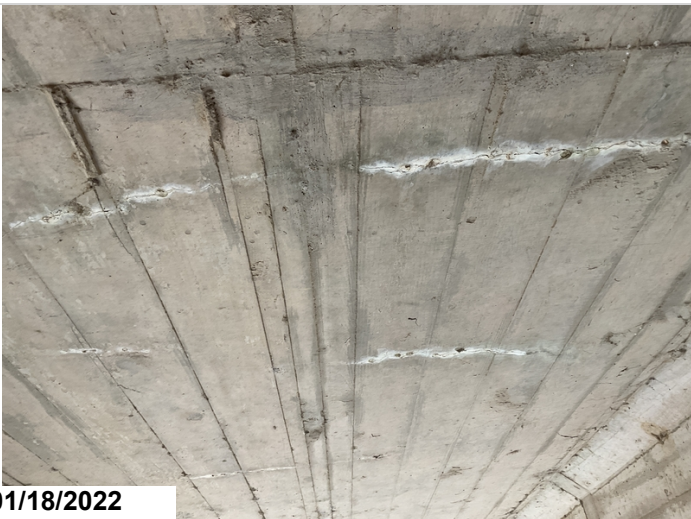
Typical efflor cracks to soffit @ all spans.
