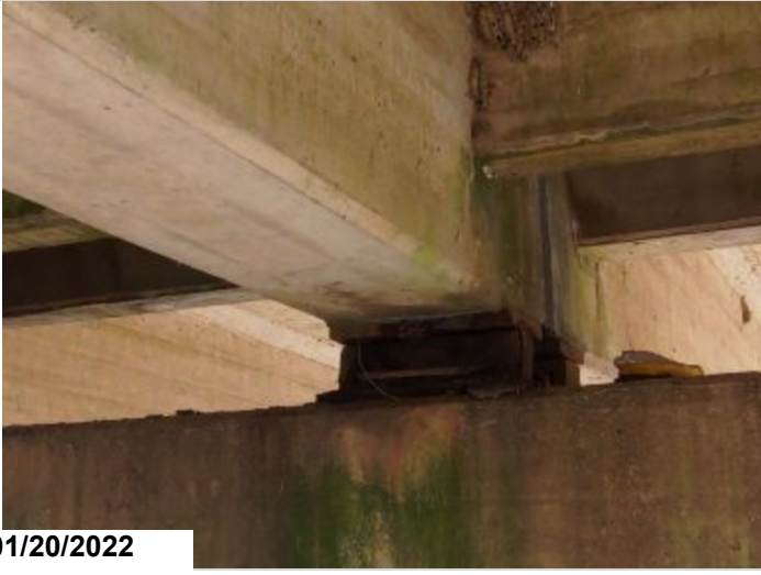
Missing anchor bolt to Girder 1 backside of Bent 1.
