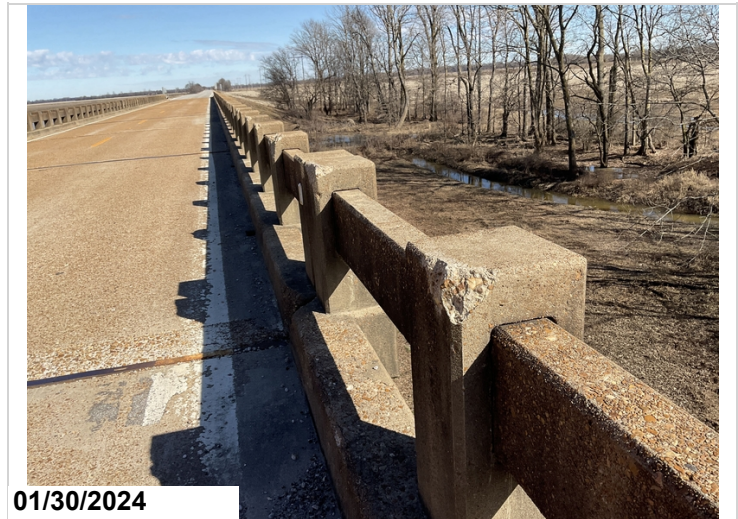
Typical spalls to tops of girders.(#3)
