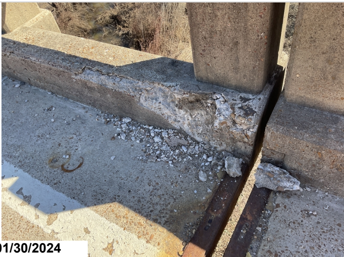
Spalls to Right curb @ beginning of Span 6.(#3)
