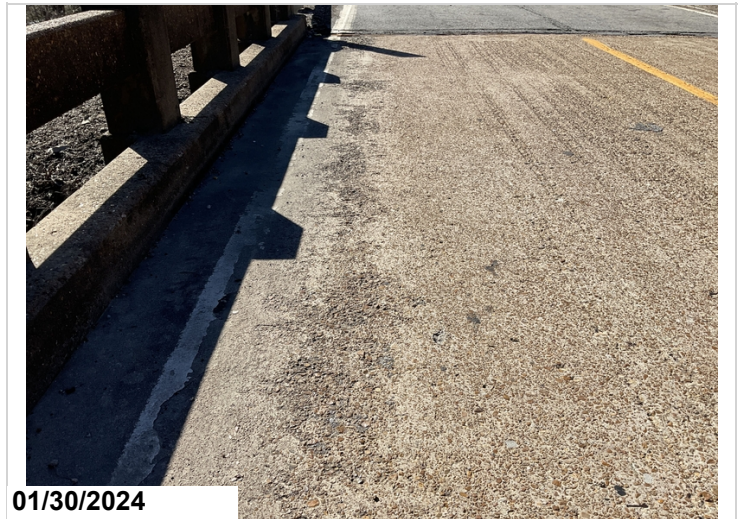
Moderate abrasion to deck in Right lane @ Span 1.(#3)
