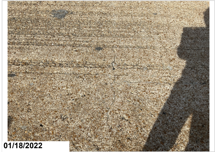
Typical cracks to deck @ all spans.
