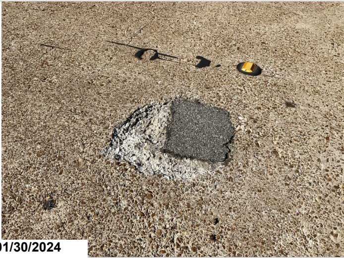
Spall with rebar exposed with s/l to deck @ Span 1.(#3)
