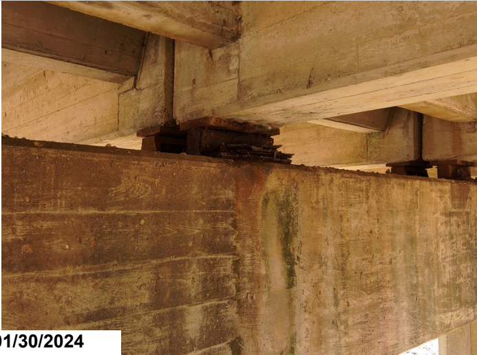
Typical rust with section loss to all bearings.
