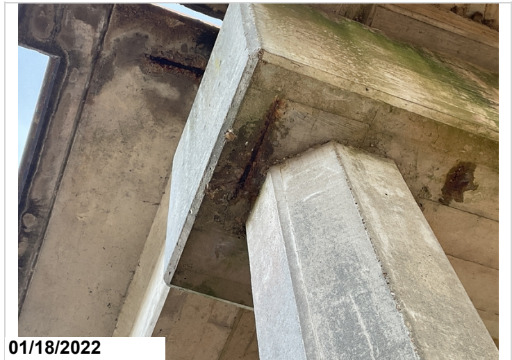
Spall with rebar exposed with s/l to Left end of cap @ Bent 6.(#3)
