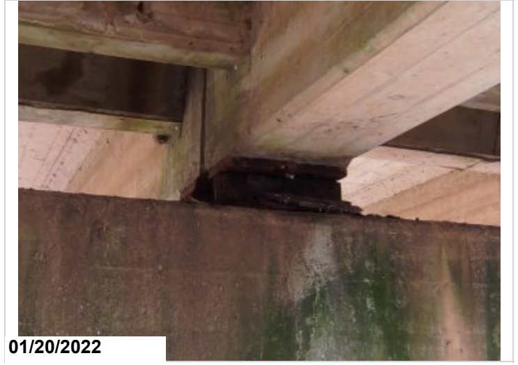
Missing anchor bolt to Girder 3 backside of Bent 1.
