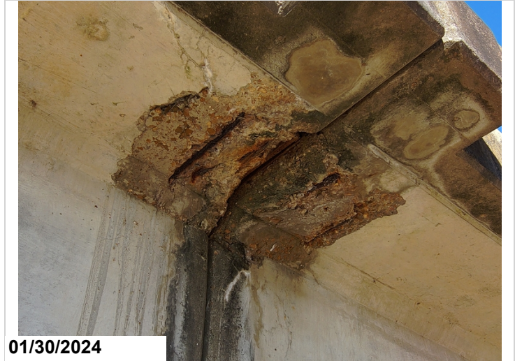
Spalls with rebar exposed with s/l to Right overhang @ Spans 9 & 10.
