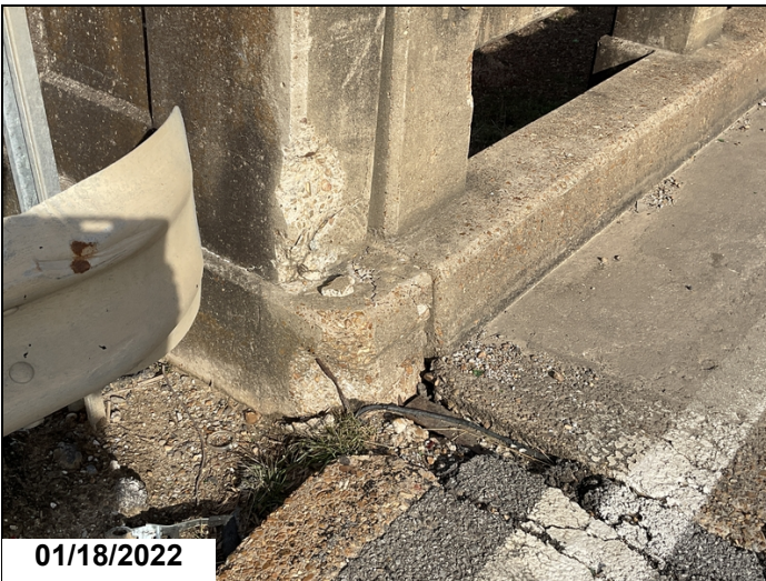
Left bridge rail posts at Spans 1, 8 and 10 have cracks and spalls to posts with rebar exposed. Span 1.
